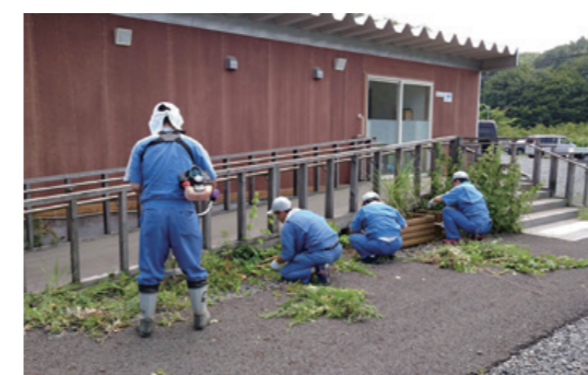
Volunteers removing vegetation by the road to make access to temporary housing easier
